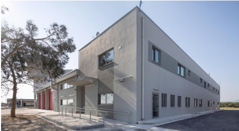
Figure 17: New rescue and firefighting (RFF) station.
