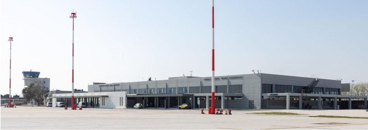
Figure 16:KVA airport, airside area.
