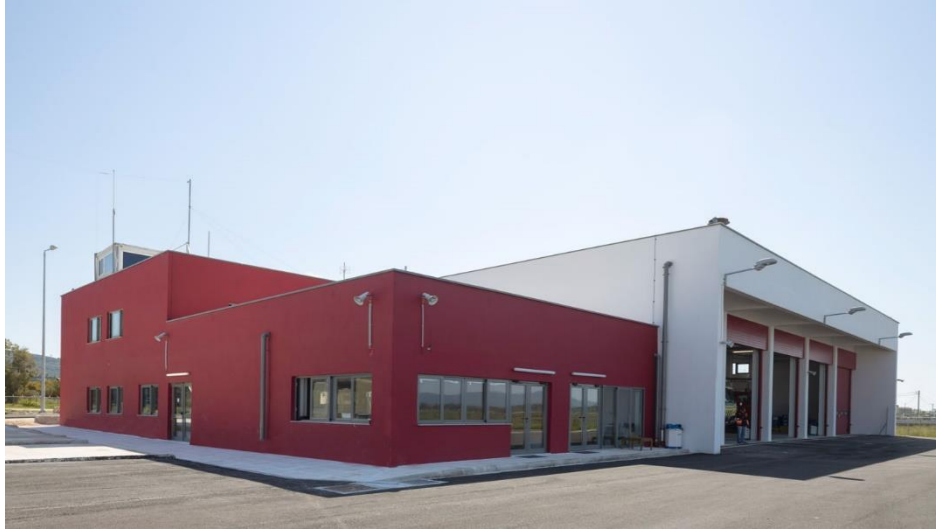
Figure 14: New rescue and firefighting (RFF) station.
