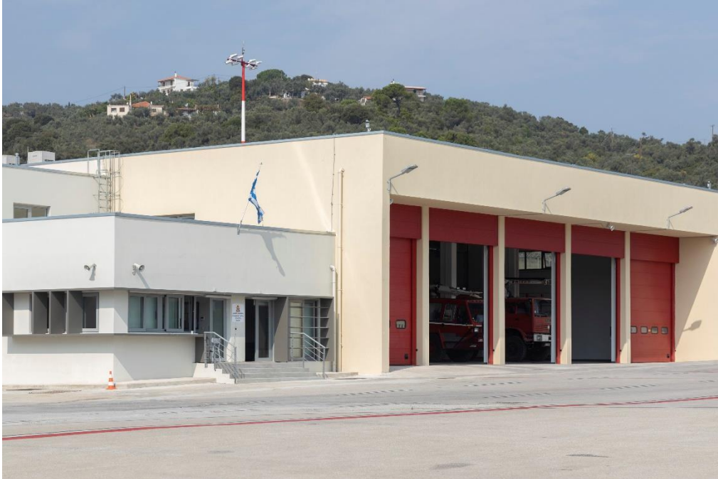
Figure 12: New RFF building.
