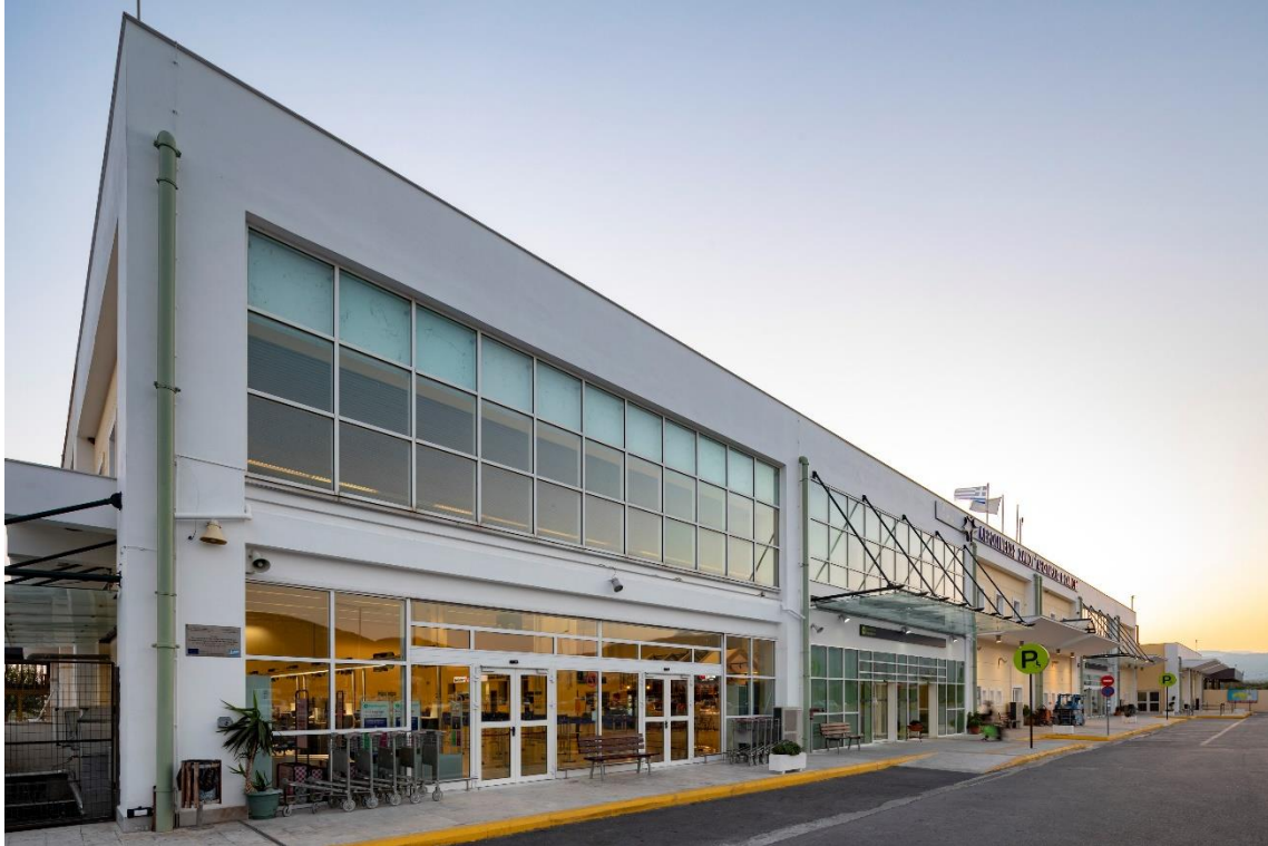
Figure 15: Terminal landside area façade..
