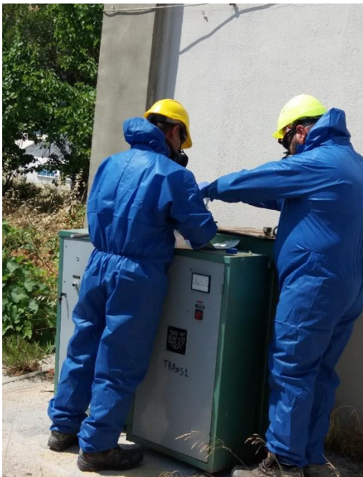
Figure 27: Sampling of PCB containing devices by specialized personnel, at MJT airport.
