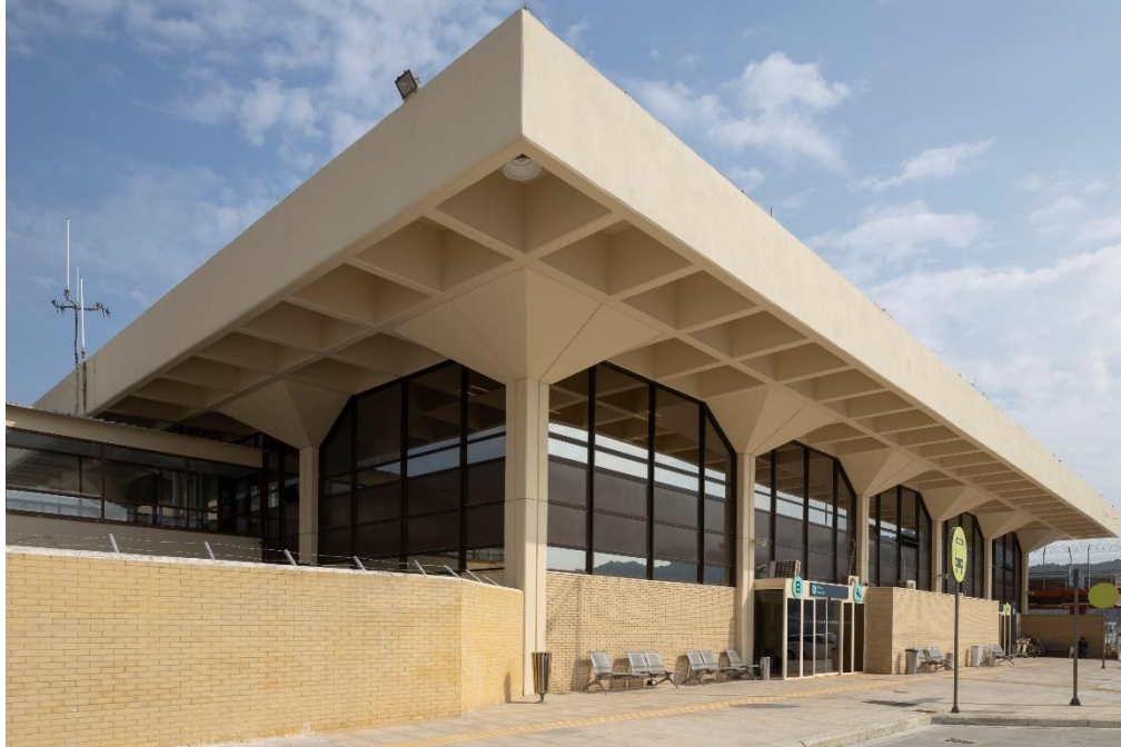
Figure 10: Terminal T1 landside façade.
