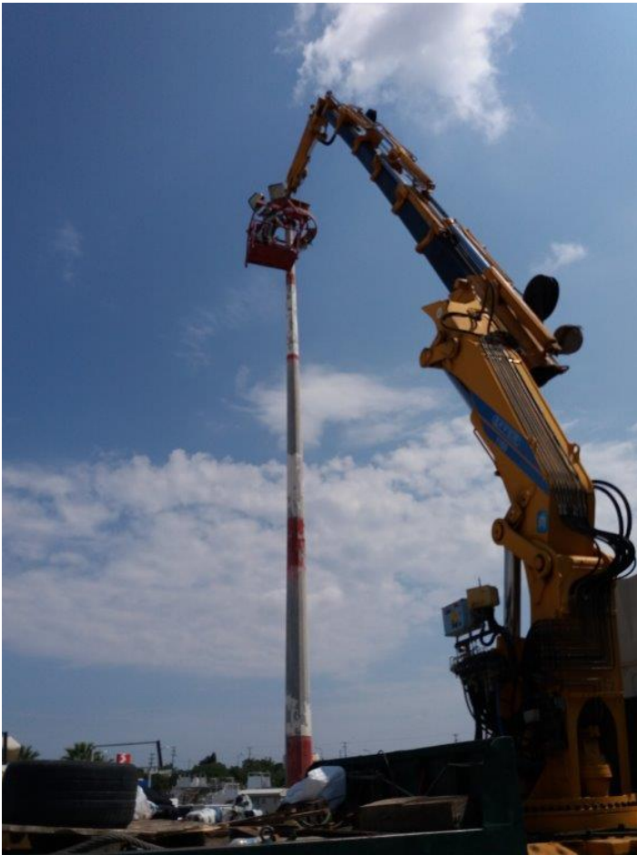
Repair of apron high mast
