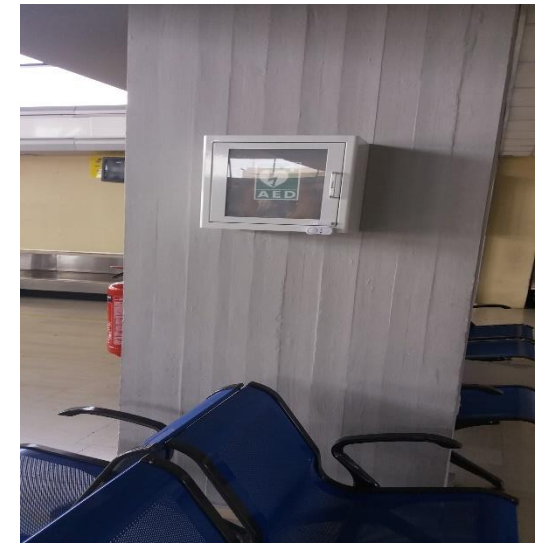
Installation of Defibrillator
