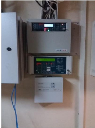
Installation of Fire Alarm System
